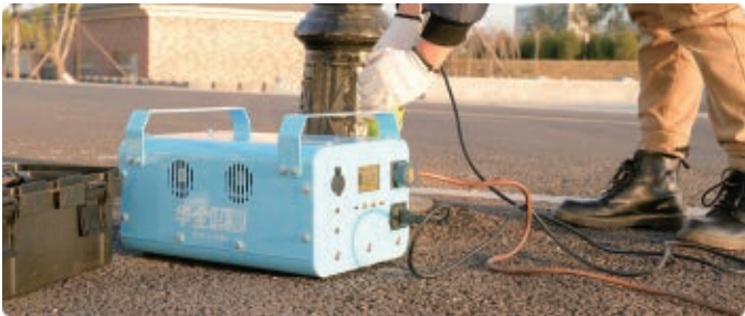
户外施工/outdoor construction
